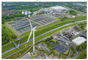
flow management rely on the optimal combination of distinct uses and sources of energy: power production from sewage sludge, sewage gas, solar panel, wind turbine; solar supported thermal drying of sewage sludge; and underway heat recovery from wastewater effluent and production of renewable e-fuel.
